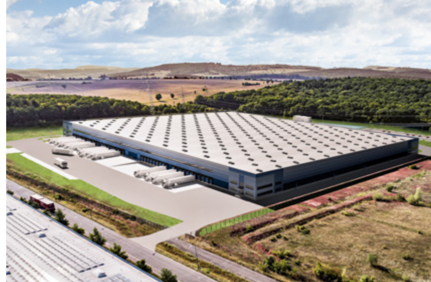
The new platform, located in Kaiserslautern, scheduled to come into service in early 2021, will cover an area of over 40,000 sq.m.
