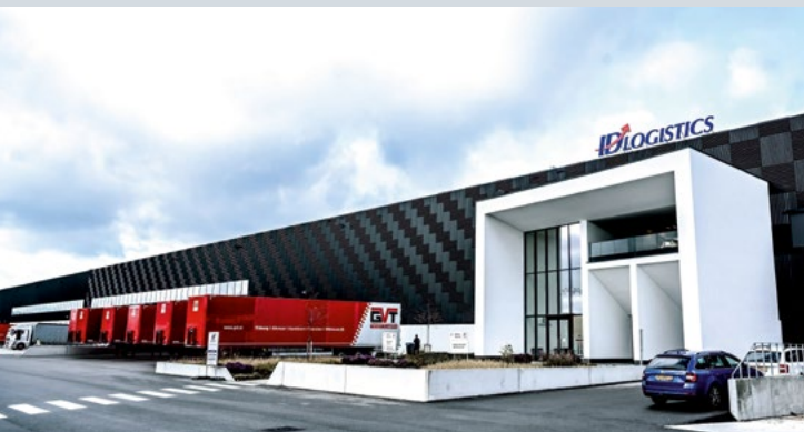
55,000 sq.m dedicated to electronics with a strong focus on e-commerce, at the Etten-Leur site (ID Logistics Benelux).
